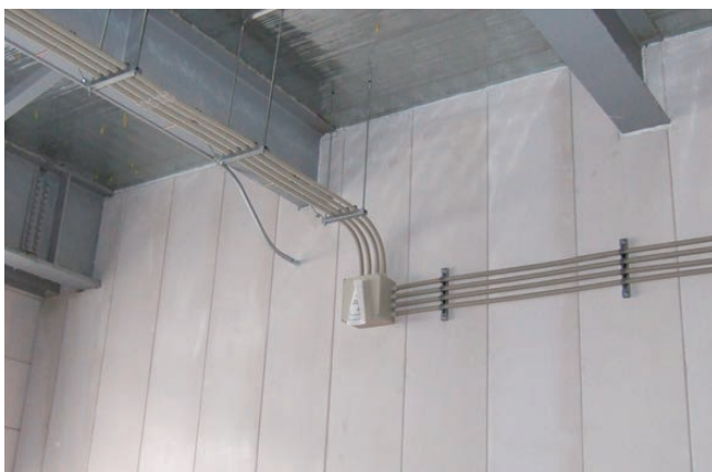
Straight conduits allowing neat installation.
