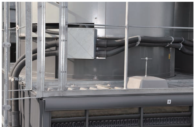
Easy installation at limited spaces where bends are required, due to its flexibility.
