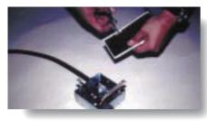
1. Cut the sheet to precise dimensions for insulation.
