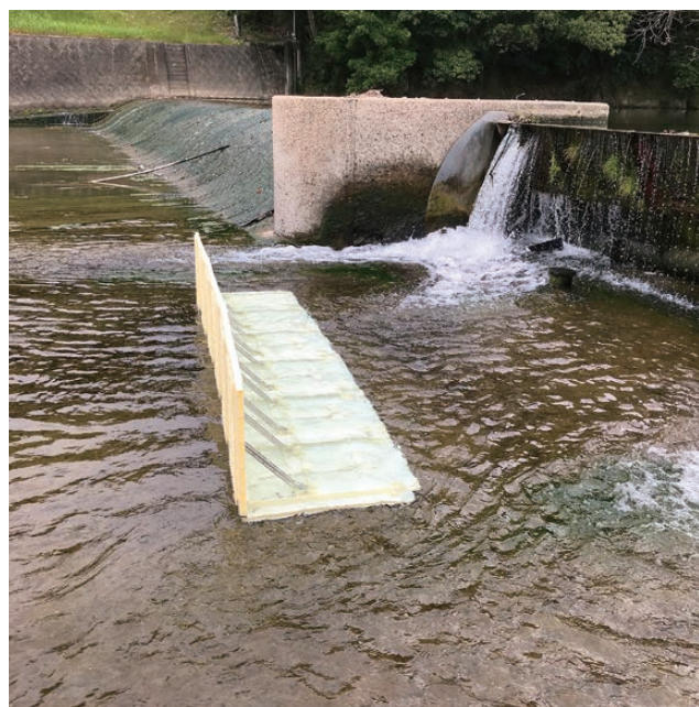
Figure 5 Field verification in Satsumasendai City.
