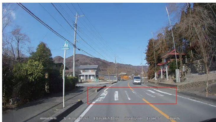
Figure 6 Examples of road marking with reduced visibility.
