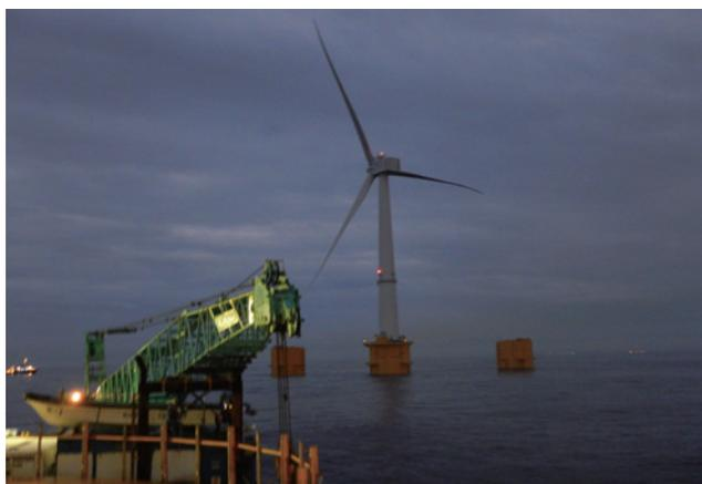
**Figure 8 The cable laying to the offshore wind turbine (7 MW class).**
