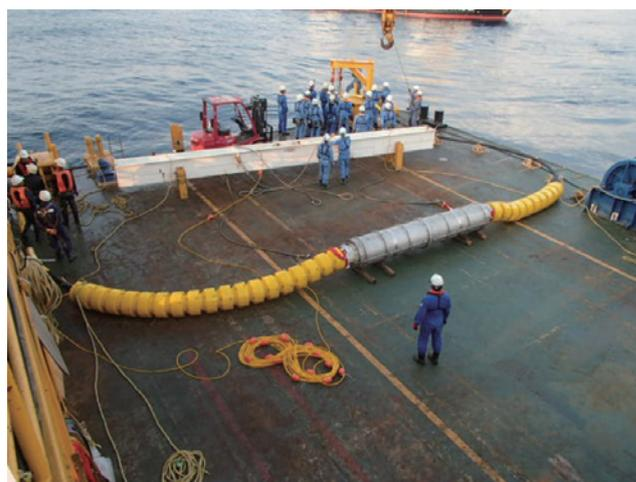
Figure 5 Appearance of the submarine joint.
