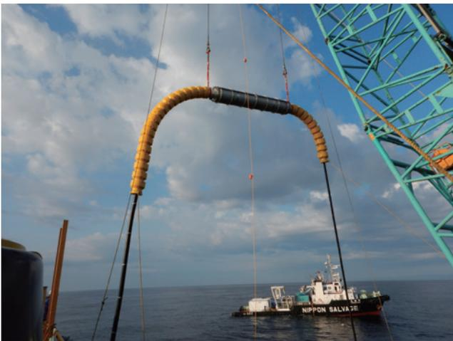
Figure 10 Submarine joint laying.
