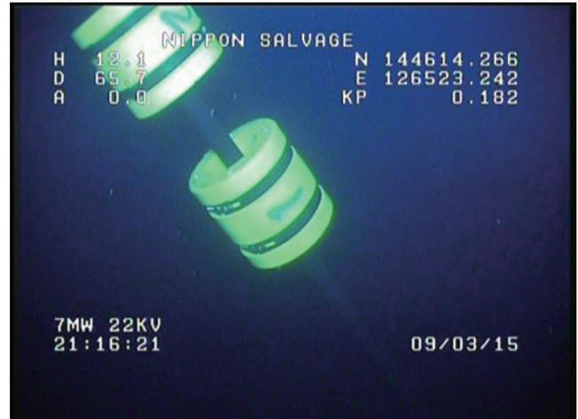
Figure 12 Line shape confirmation by ROV.
