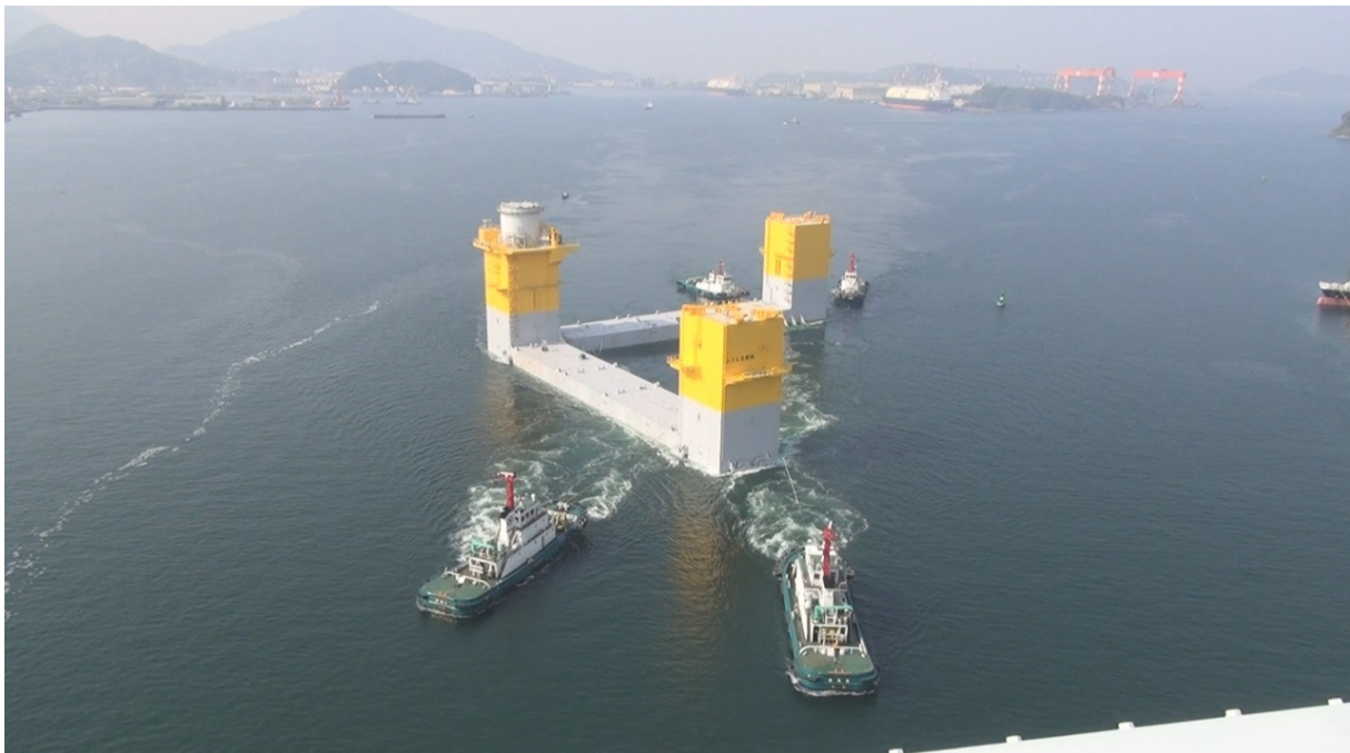
Towing the three-column semi-sub at Nagasaki port
