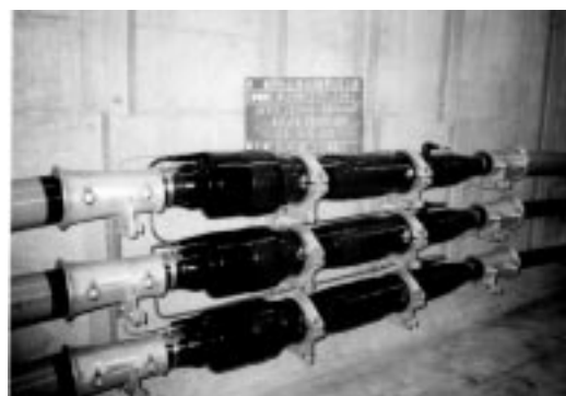
写真5 RMJ組立て状況 View of RMJ on site
