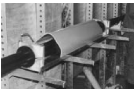
写真3 絶縁筒の収縮現場 Assembly of cold-shrinkable joint on cable
