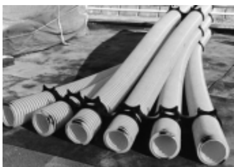
写真8 管崩し施工例 Transition from bundle layout to array layout
