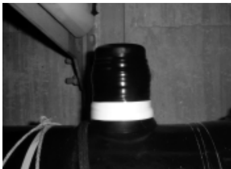
図4 活線採油コネクタの直線接続部への取り付け例 On-line sampling connector installed on a joint box for oil filled cable line
