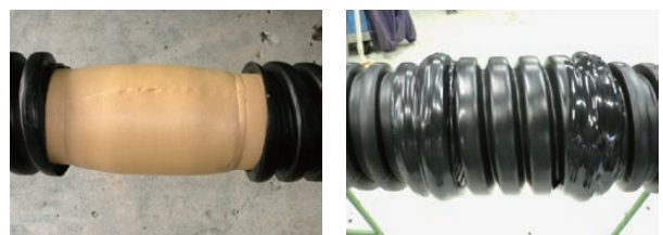
図13 継手の施工 Installation of pipe fitting.
