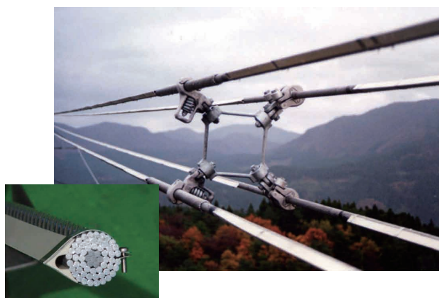
図34 模擬着雪の取り付け状況 Installed wind-load fixture to simulate snow accretion.
