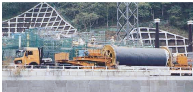
図2 特殊車両での長尺布設 Laying of long-length cable using special-purpose vehicle.
