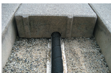
図2 灌水パイプ収納状況 Accommodation of sprinkling pipe.
