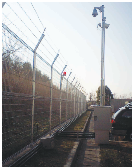
図6 施工例2 Installation example (II).
