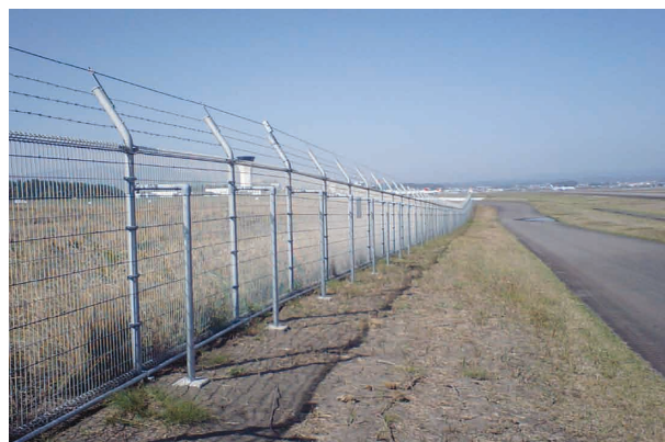
図2 施工例1 Installation example (I).
