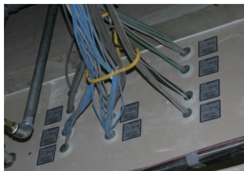
図4 プチロク壁貫通部施工例（福祉施設） Example of PUCHIROKU installation (in welfare facility).
