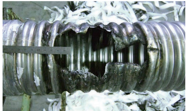
図8 内管コルゲート管の損傷の様子 The appearance of the damaged inner corrugated pipe.
