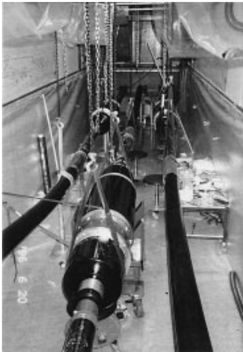
Photo 1 420-kV prefabricated joint
