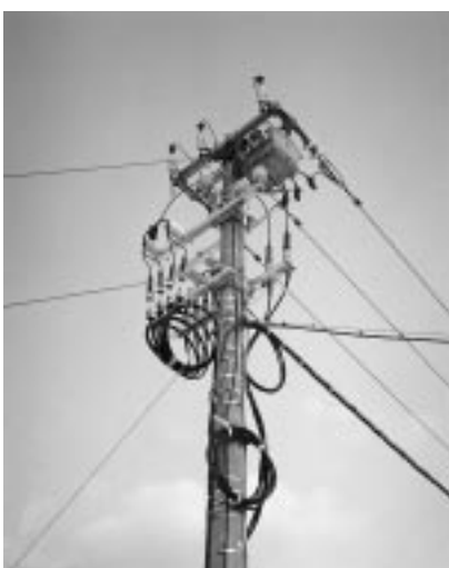
Photo 4 Outdoor exposure test (heavy pollution area)
