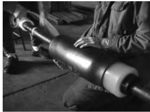
Photo 1 Assembly of rubber molded sleeve for CSJ onto bonded cable
