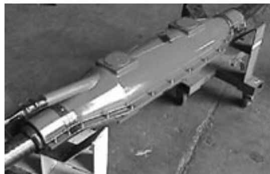
Photo 3 Appearance of the completed 110-kV CSJ
