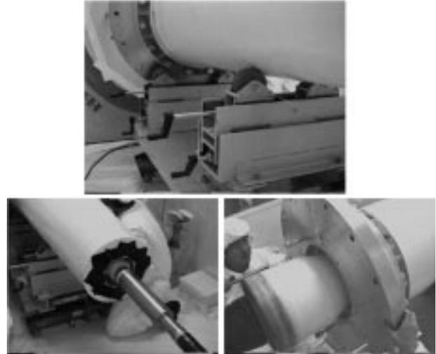
Photo 5 Techniques for laying the horizontal gas-immersed sealing end
