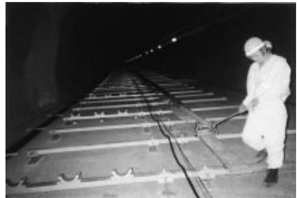
Photo 3 Laying cable in the tunnel
