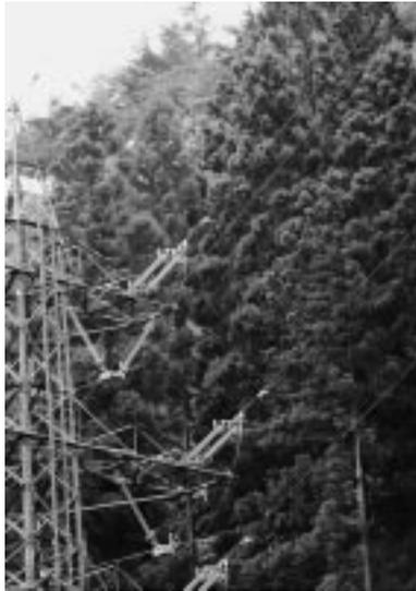
**Photo 4 Composite insulator installed on working transmission line**
