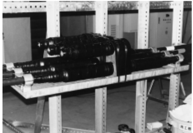
Photo 2 Appearance of installed Y-branch joint
