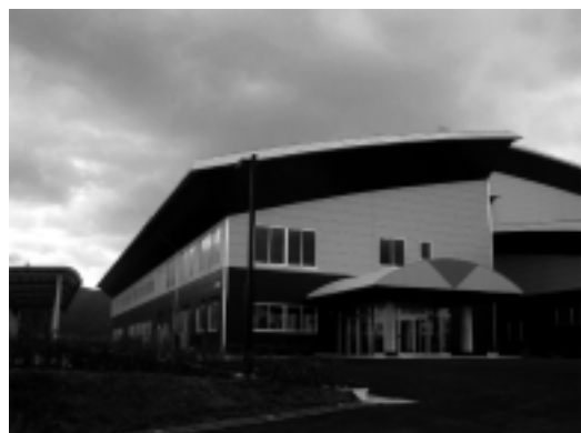
Photo 1 View of Chouyo martial arts gymnasium (main building).
