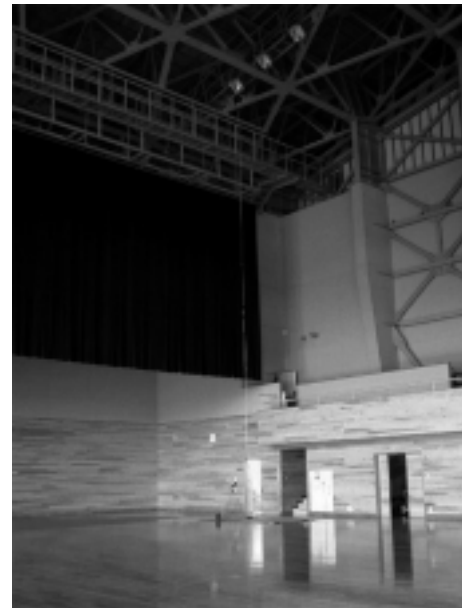
Photo 3 Measurement points in the main building.
