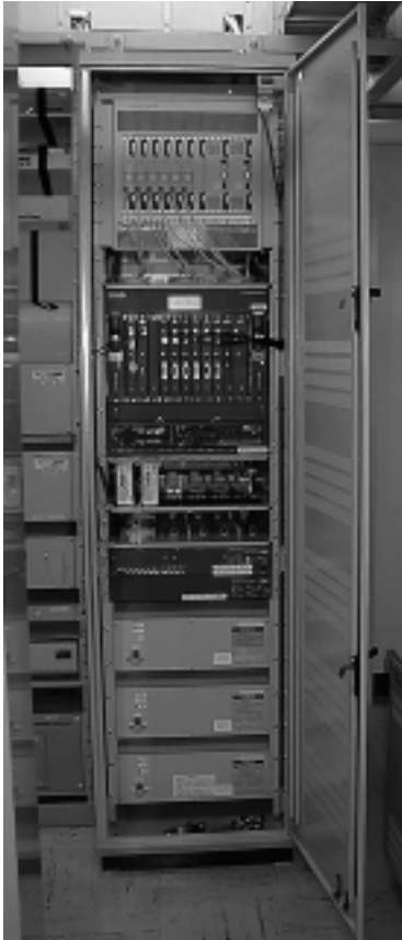
Photo 1 HE center equipment.
