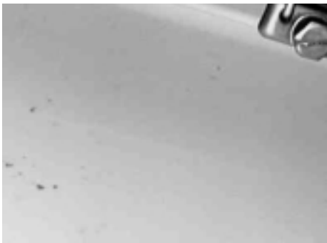
Photo 3 Dew condensation eliminated after installation of DryKeeper.
