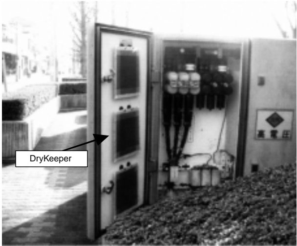
Photo 1 Field test of DryKeeper in a cabinet for high-voltage use.
