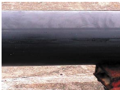
Photo 9 Appearance of outer sheath after laying test.
