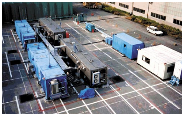
Photo 1 Appearance of treatment facility.
