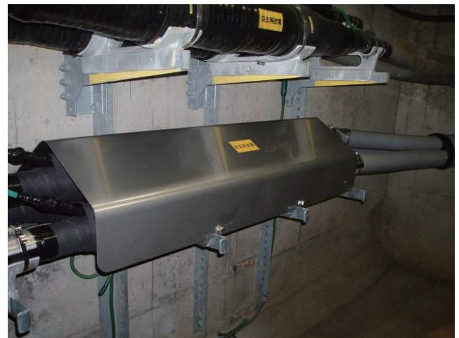
Figure 4 View of assembled ERJ with protection cover.
