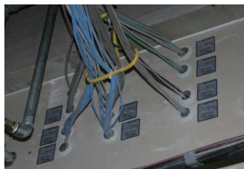
Figure 4 Example of PUCHIROKU installation (in welfare facility).
