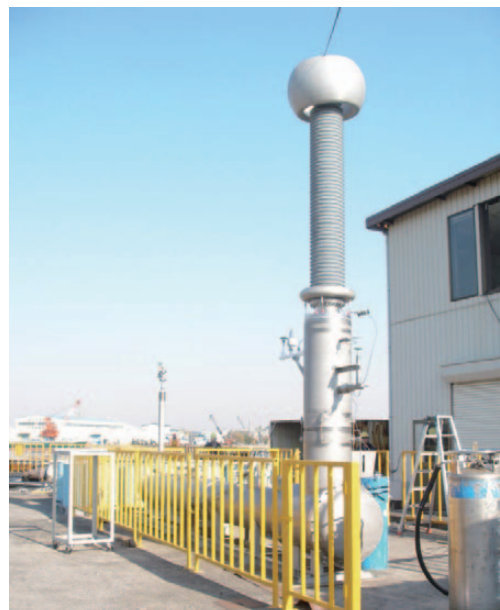
Figure 10 Termination for 275 kV HTS cable.
