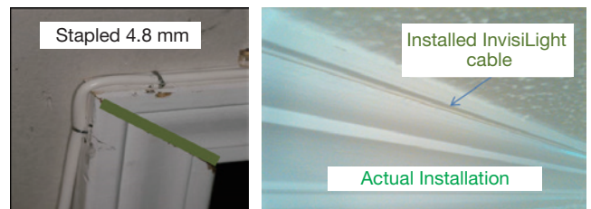
Figure 3 Examples of the deployed ultra-bend-insensitive single-mode optical fiber in the existing buildings.
