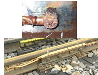
Rail bond made using copper thermite
