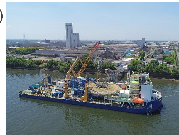
Loading submarine cable onto a barge
