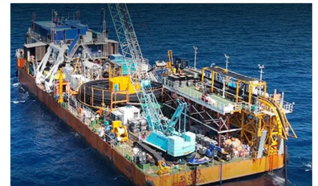
Loading the submarine water supply pipes onto a barge
