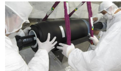
Underground cable installation worksite
