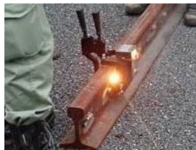
Welding using copper thermite
