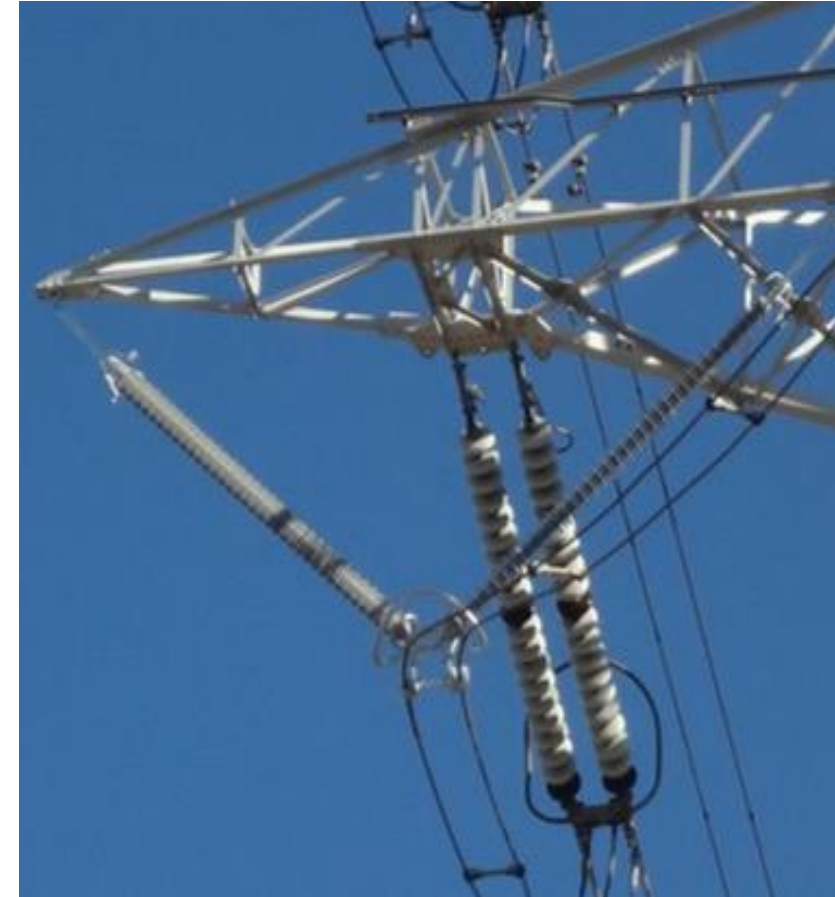
V-string assembly for jumpers
