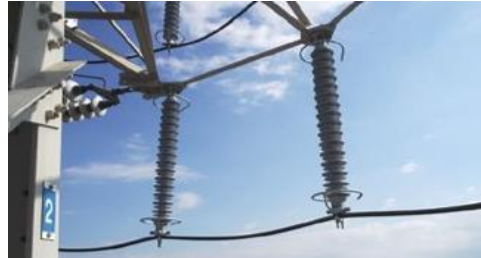
I-string assembly for jumpers
