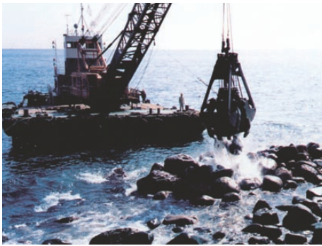
Excavating a trench
