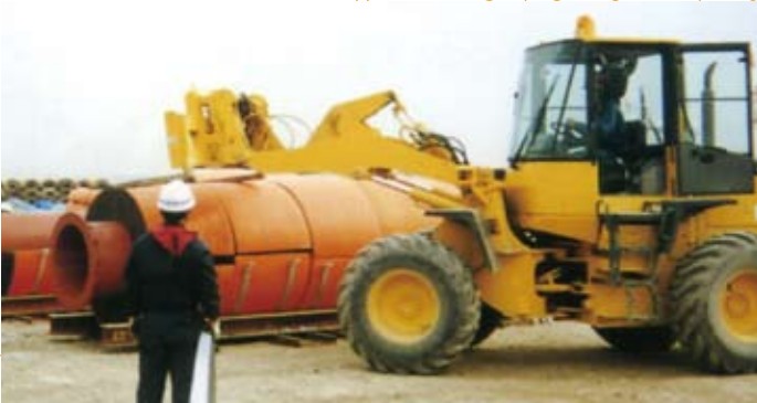
3 Wooky (upper half) is overlaid. The size is designed to be a little tight to prevent coming off. Press it down to fit properly.
