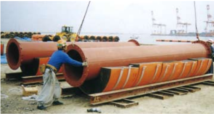
2 Sand discharge pipe is laid down.
