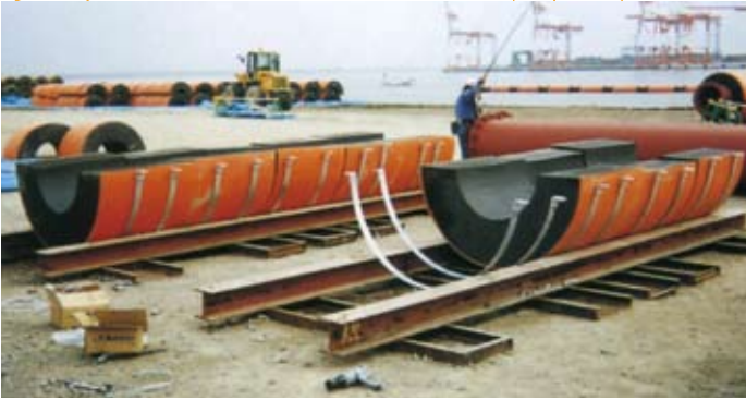
1 Metal cramp and Wooky (lower half) are arranged.
