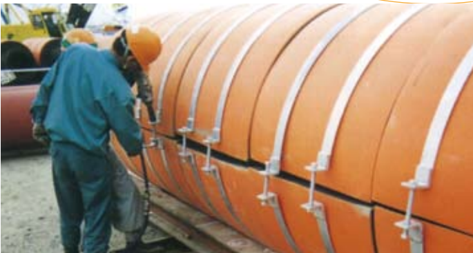
4 Fasten the bolt firmly so that the metal cramp sinks somewhat into the surface.
