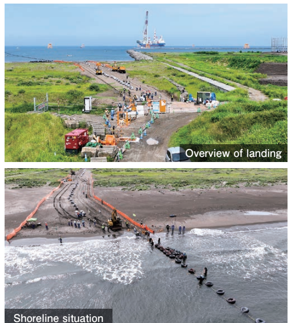
Figure 4 Landing of the submarine cable.
