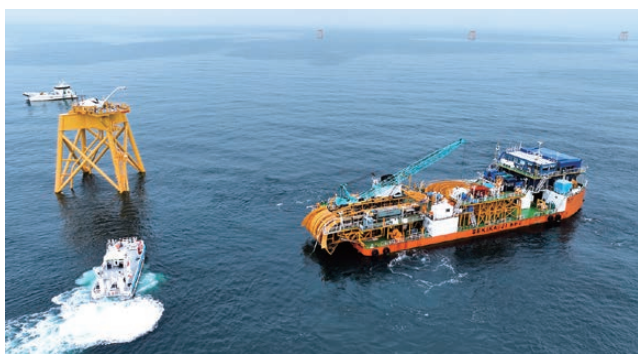
Figure 6 Laying of the submarine cables to the wind turbines.
